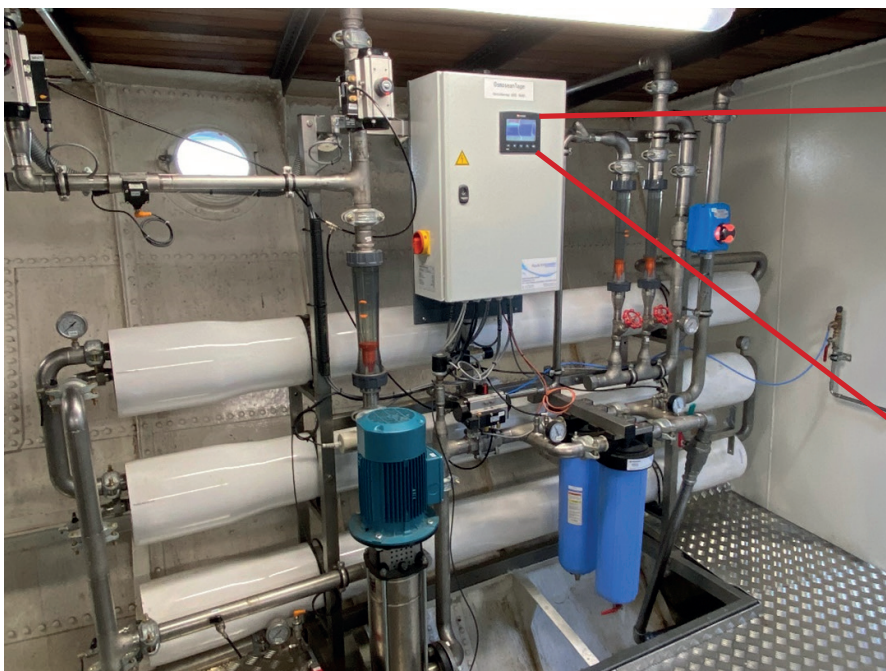
V430 PLC for controlling the reverse osmosis plant for the water production of the «City of Rapperswil» of the ZSG.
