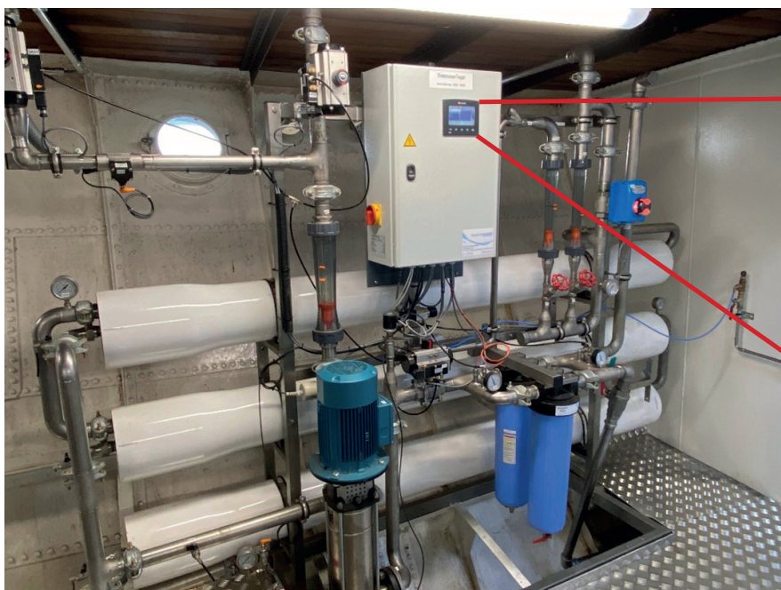
V430 PLC for controlling the reverse osmosis plant for the steam generation of the «Stadt Rapperswil» of the ZSG.
