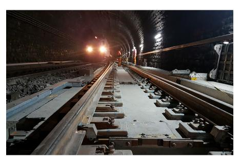
The ballast terrace is replaced by a concrete base. Extra-wide trains would endanger safety on the construction site and must be stopped.
