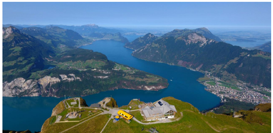
The water supply at the mountain restaurant Klingenstock perfectly works thanks to the CMS-10R.
